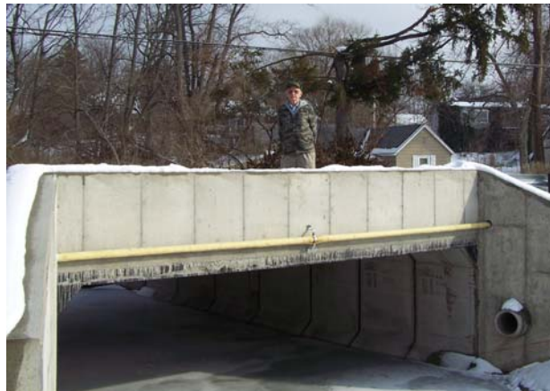
Lifelong Morgan Place resident Cecil Morgan is shown at the Englewood Drive bridge which was replaced in 2010
